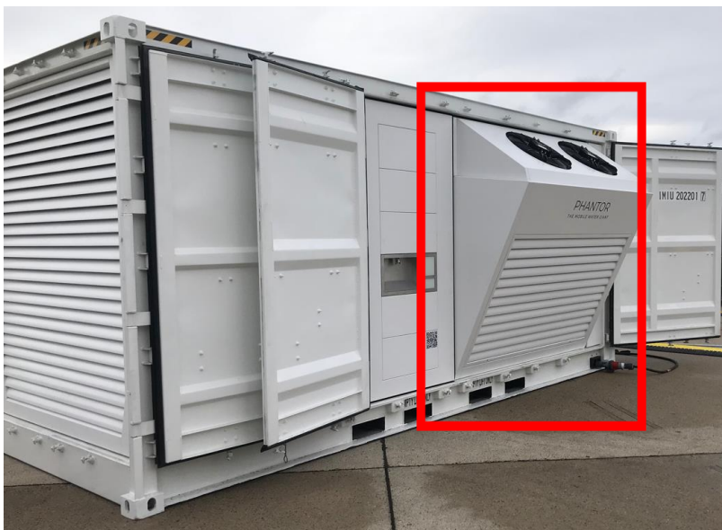
Figure 13: Condenser left in extended state
