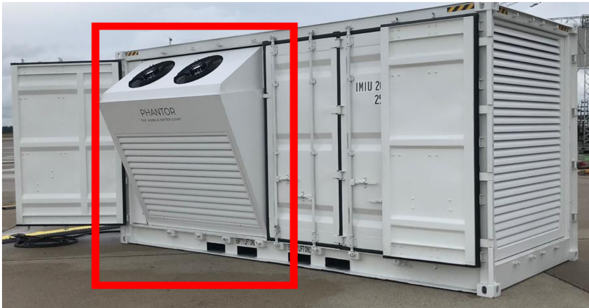
Figure 12: Condenser right in extended state
