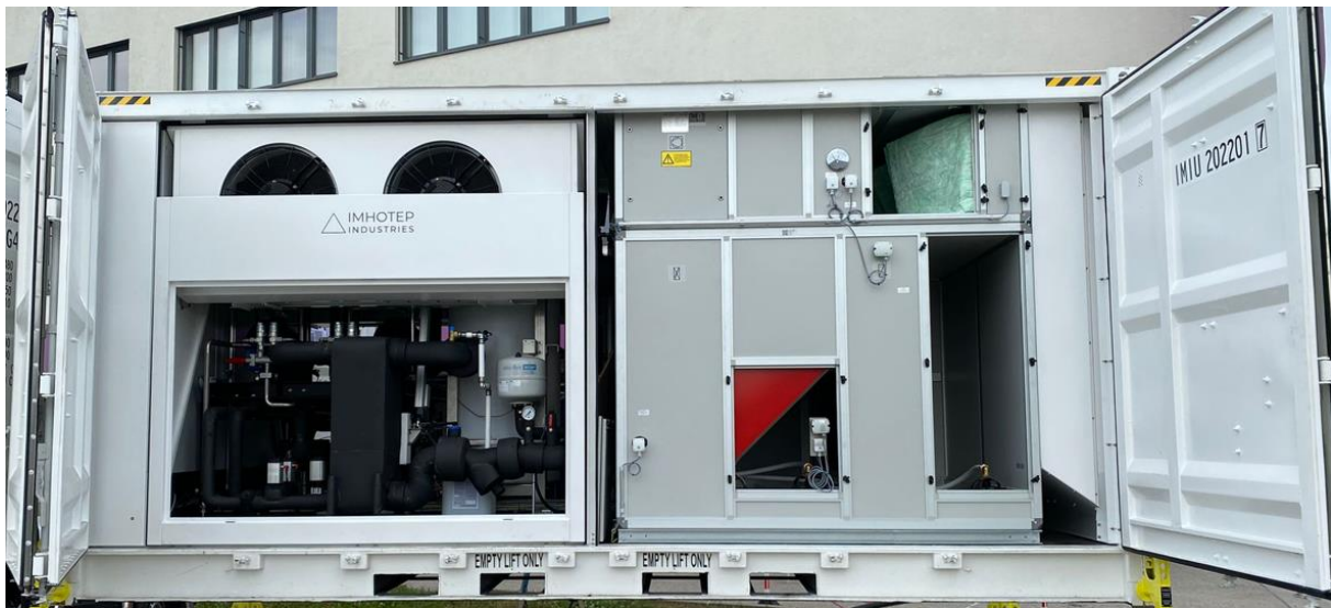
Figure 16: Phantor 6000 with open inspection ports
